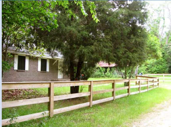
New board fence along front road
