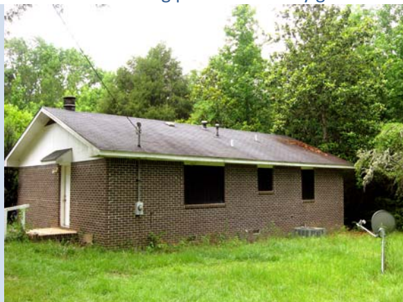
Back yard showing HVAC unit and satellite dish. Small pond is farther to the right.
